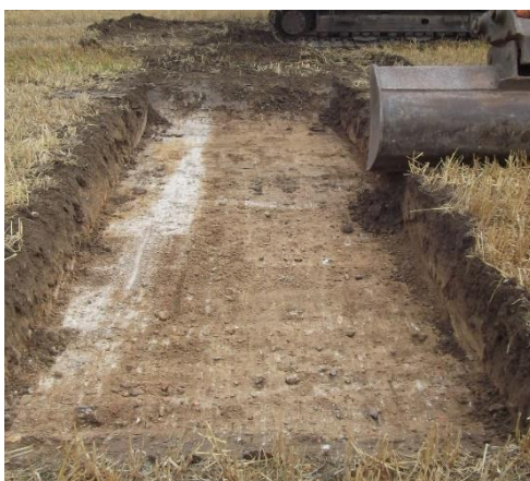
Figure 7: Trench 4 after the initial mechanical excavation
